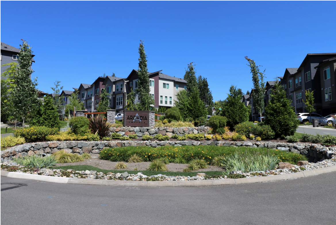
Arcadia Terrace Townhomes - 91 Units
